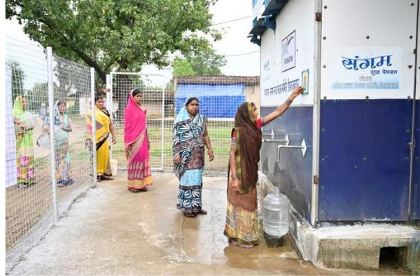
Considering the challenges faced by communities in these two villages to get clean and safe drinking water, JSPL Foundation installed community-based safe drinking water system UV treated Water ATM in village Jhinkabahal in 2016 & village Kasdol in 2019. Besides Four solar-based drinking water systems were also established in village Tehlirampur, Regaon, Manjhapara in collaboration with CREDA (Chhattisgarh Renewable Energy Development Authority).
