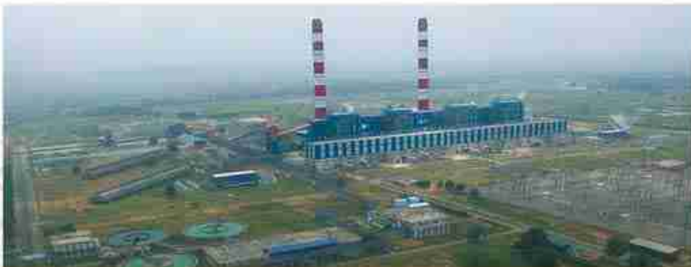
Aerial view of the 1000 MW mega Power Plant, Raigarh
