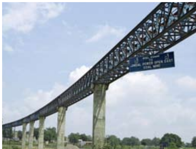
7 km long Conveyor Pipeline
