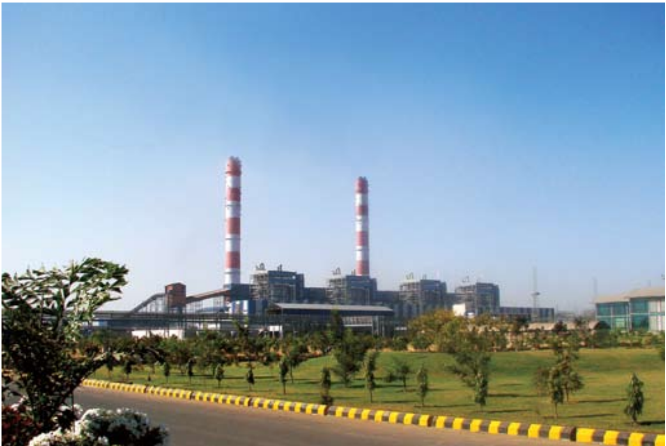
1,000 MW Thermal Power Plant at Tamnar, Raigarh
