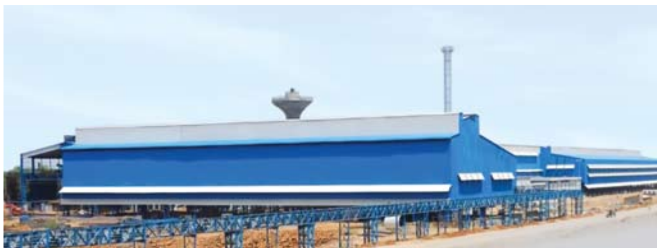
Overview of Wire Rod Mill at Patratu, Jharkhand
