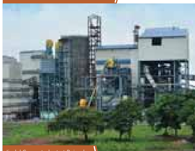
Jindal Cement plant at Raigarh
