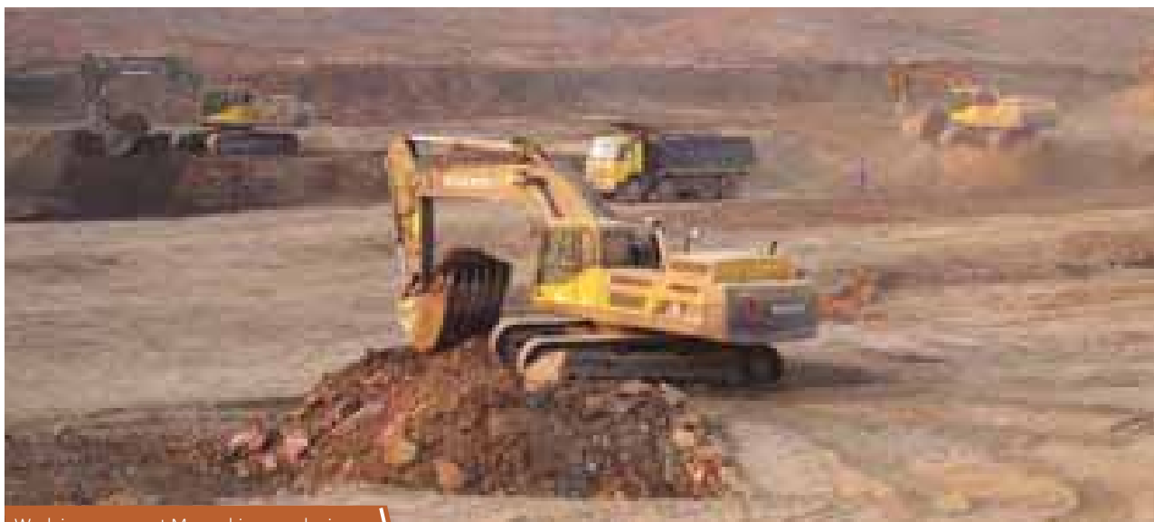
Work-in-progress at Mozambique coal mines
