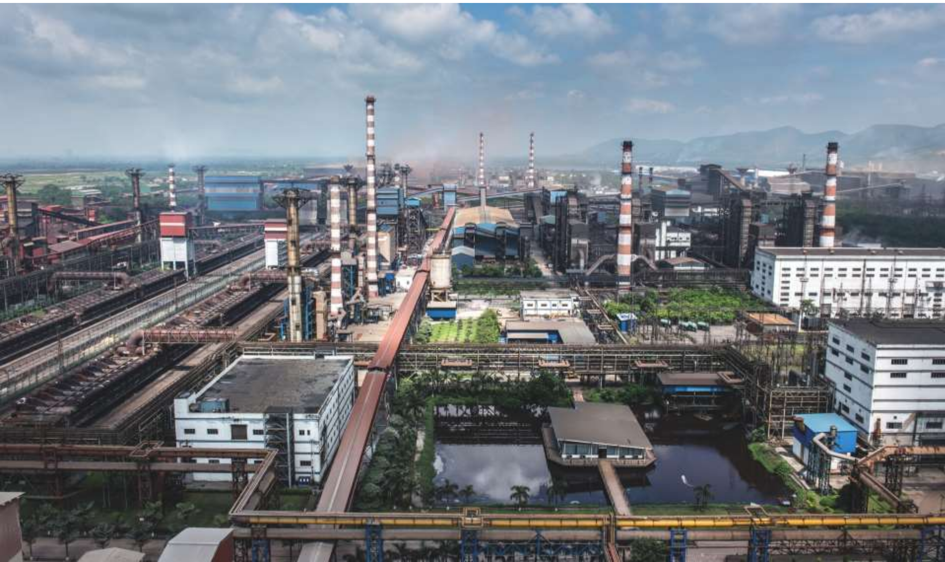
Aerial View of Raigarh Plant
