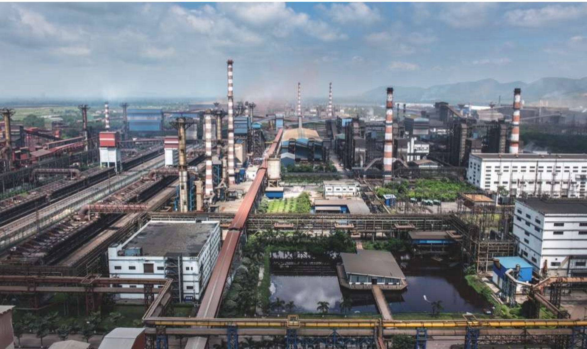
Aerial View of Raigarh Plant
