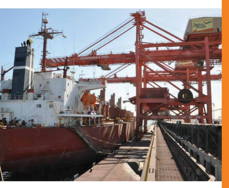
Jindal Shadeed has a 600 mtrs long captive jetty with ship loaders/un-loaders to handle import and export activity. It can accommodate large capesize vessels upto 180000 mt dwt with its draft of 19 mtrs.
